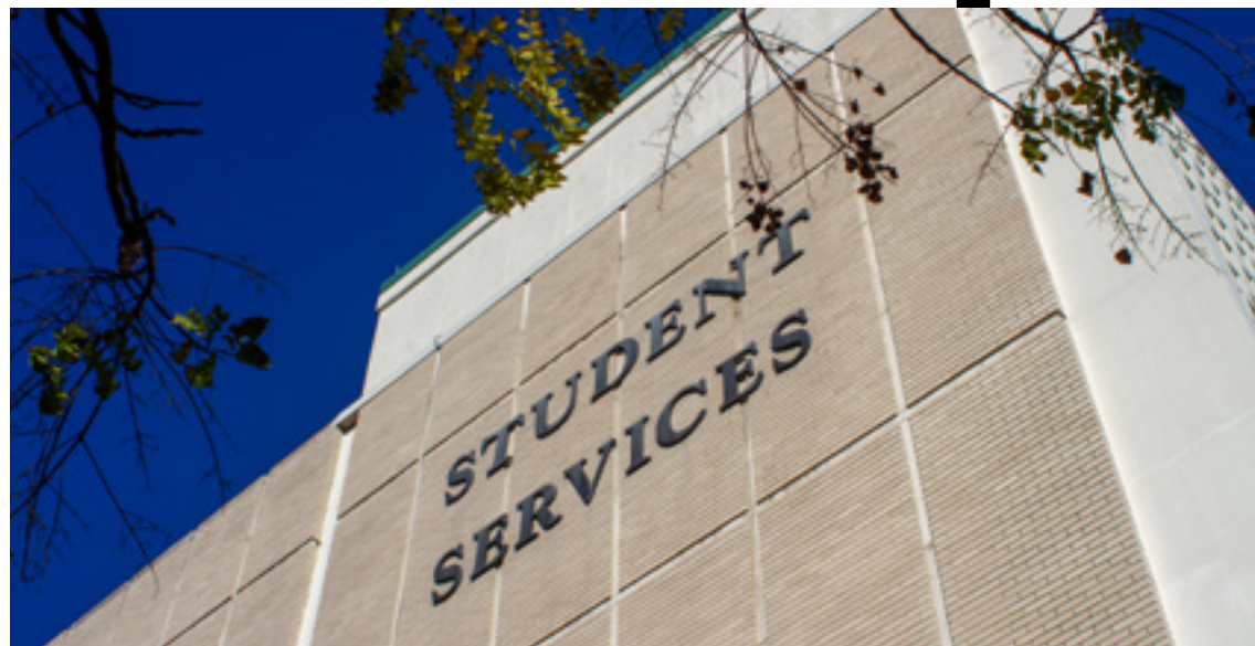
Royal Aire will replace multiple air handling units to improve ventilation in the basement and first, second and fifth floors. ORACLE PHOTO/ALEXANDRA URBAN
